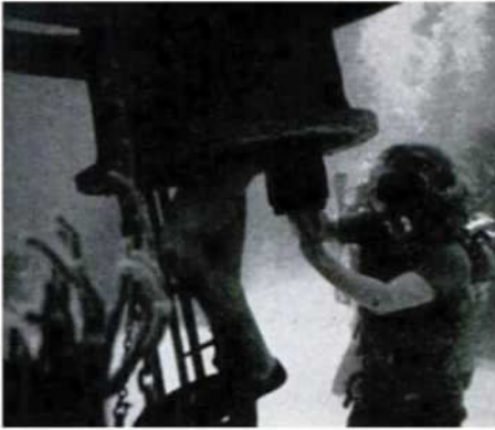
Paying a visit beneath the sea, Dr. von Braun approaches entrance at bottom of cylindrical sea lab, made of rubberized fabric and inflated with air.
